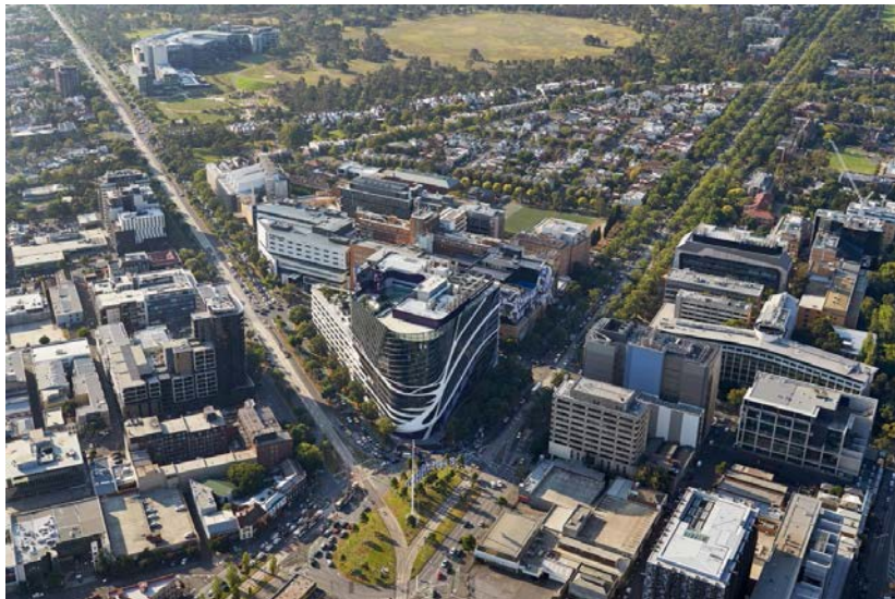
Photo by Peter Bennetts, courtesy of Plenary Group
